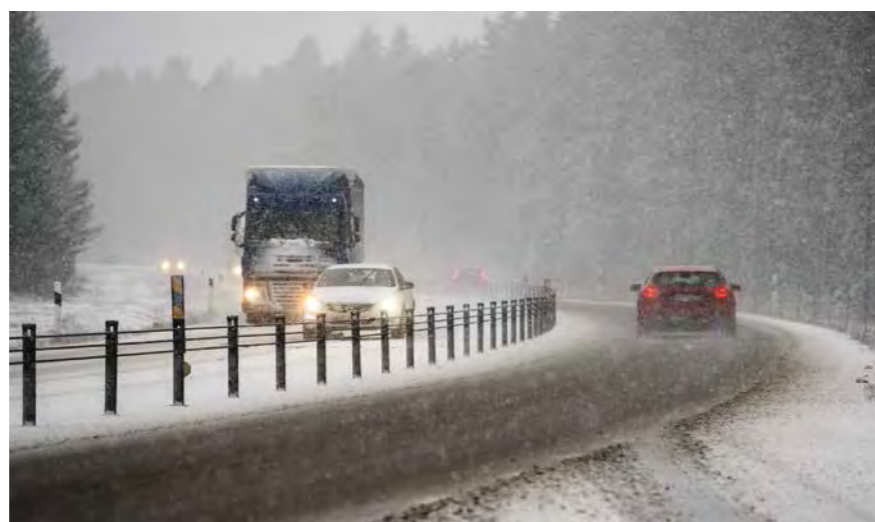
8. Una strada con barriera mediana (photo credit: Kerstin Ericsson, Trafikverket - Swedish Transport Administration)
