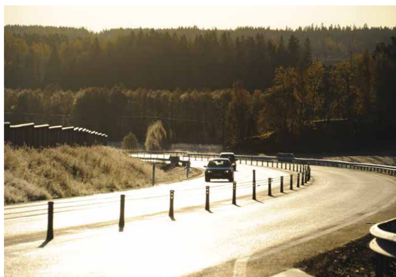
3. Una strada con barriera mediana (photo credit: Kerstin Ericsson, Trafikverket - Swedish Transport Administration)
